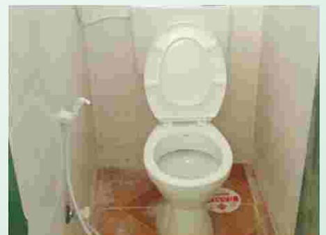
The newly built public toilets in Gaza.
